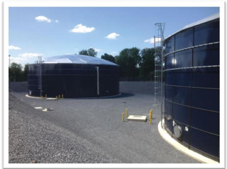
One of the biggest differentiators of CST's glass-fused-to-steel tank is its multi-step fabrication process:
